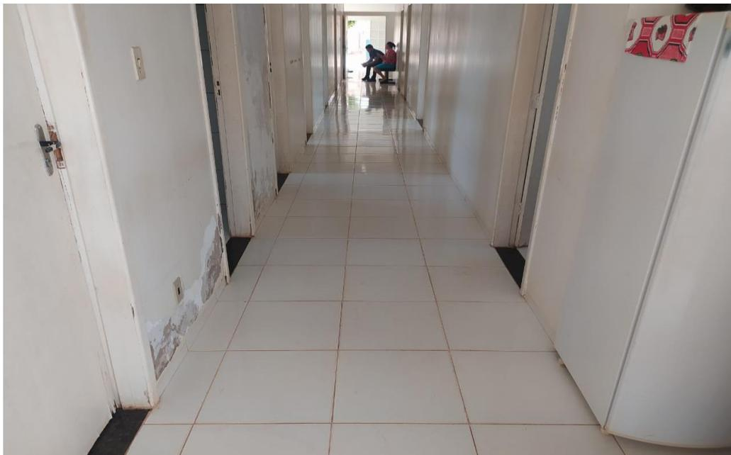
8 - FOTO – PAREDES INTERNAS DANIFICADAS - REPARAR PAREDES E EXECUTAR PINTURA GERAL, SUBSTITUIR FOLHA DE PORTA E INSTALAR FECHADURA COMPLETA.
